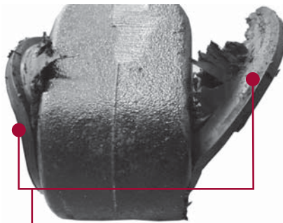
Disconnected Rubber Flange
